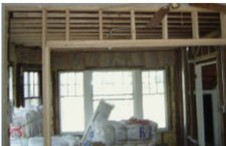
Looking into the dining room from the family room. Dining room cabinets have been removed to restore the bay window to its original size.
