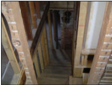
Looking down from the third floor to the second floor.
