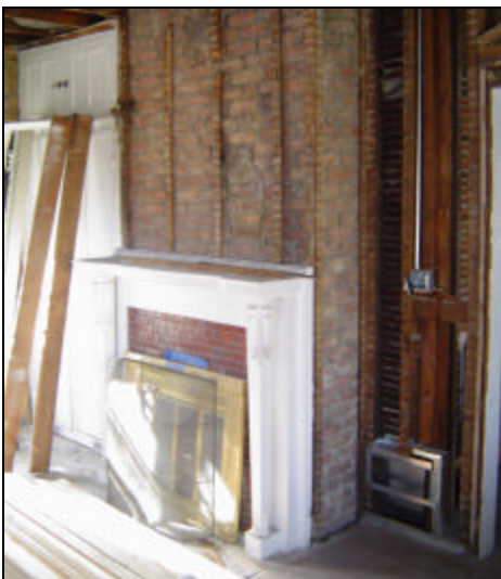
Living room fireplace with the lath and plaster removed.
